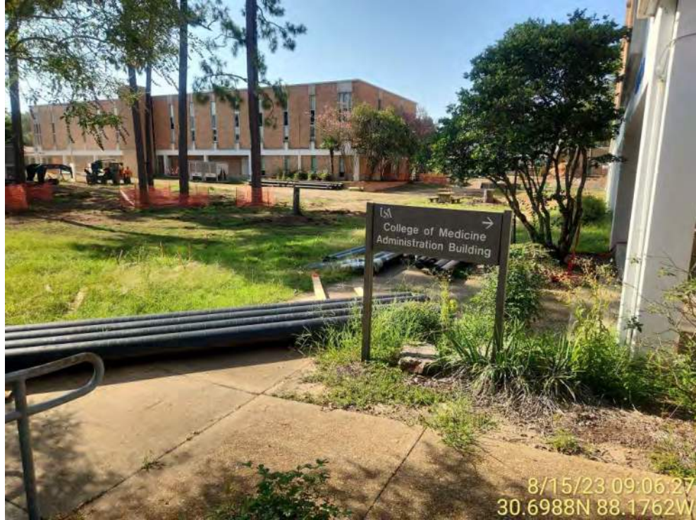
Photograph 5 – View South to Alpha South from College of Medicine Administration Building (old Alpha West)
