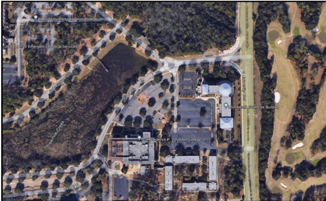
Figure 15. Parking Lots and Access Roads around the Frederick P. Whiddon College of Medicine.
