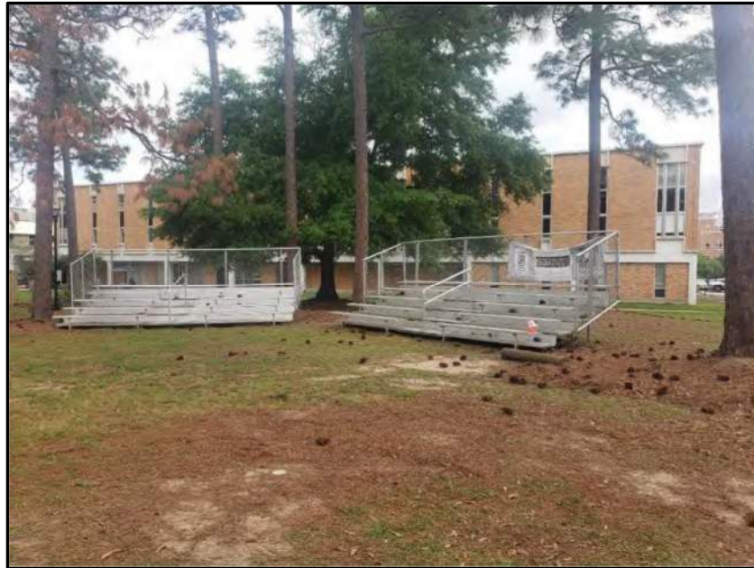
Figure 10. ROTC bleachers in inner courtyard.
