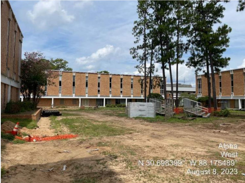
Photograph 23 – Adjacent properties to the west.
