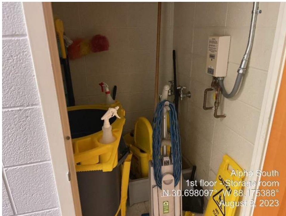
Photograph 16 – Alpha South – Janitorial Storage Room.
