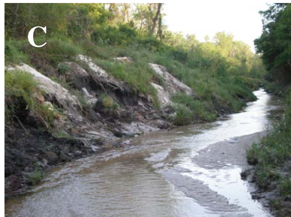
Figure 6a, 6b, 6c: Erosion occurring on the slopes of the stream.
